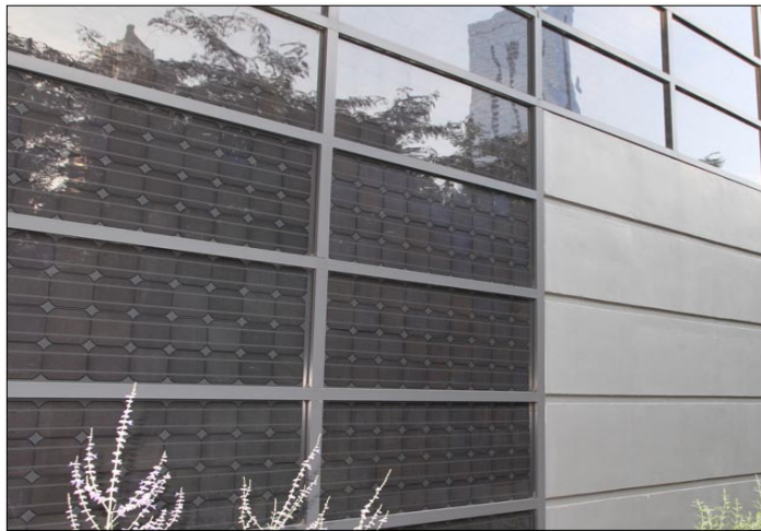
Photovoltaic panels are shown here on the Exelon Pavilions. Ryan Mikulenska
