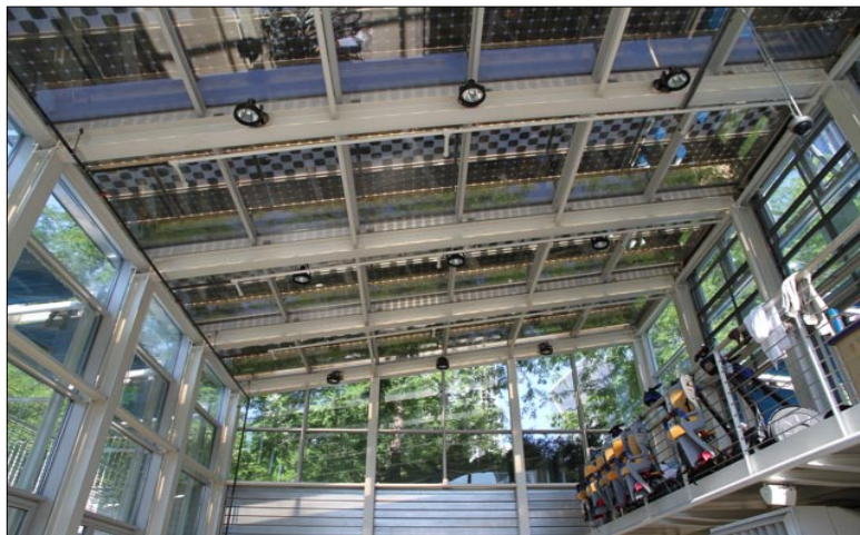
120 solar panels on the roof of the McDonald’s Cycle Center produce about 6.5% of the electricity supply required.
