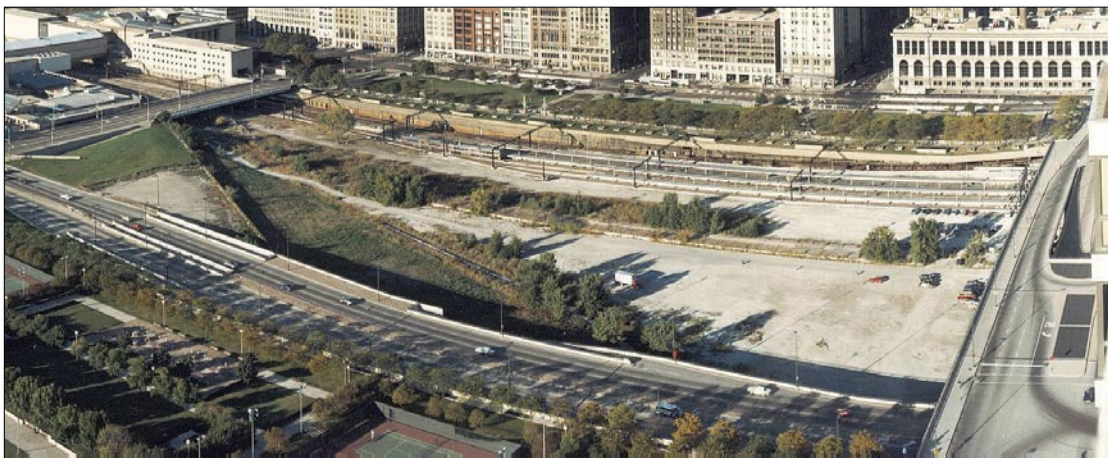
Millennium Park site before park construction began. Millennium Park Inc.
