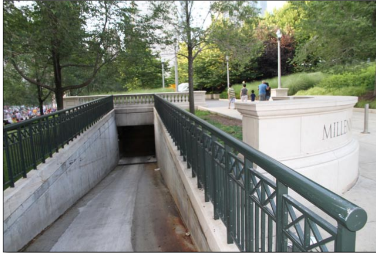
The ramp that leads to the underground trash storage facility can be seen here. Storing the trash underground helps enhance the park's smell. Ryan Mikulenska
