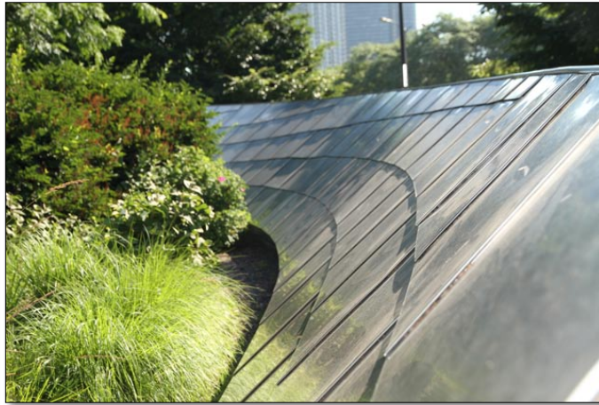
Steel plates form the exterior "skin" of the BP Bridge. Ryan Mikulenska
