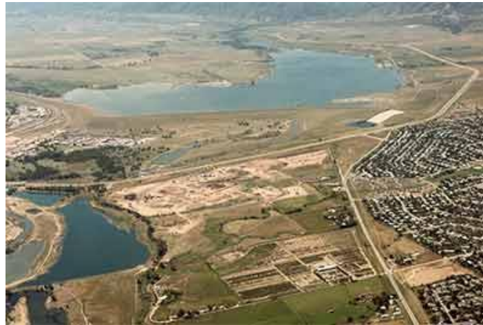
New Reservoir Construction
